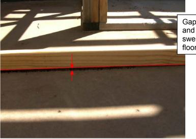
Gap between straight edge and floor indicates edge swelling in particleboard flooring
